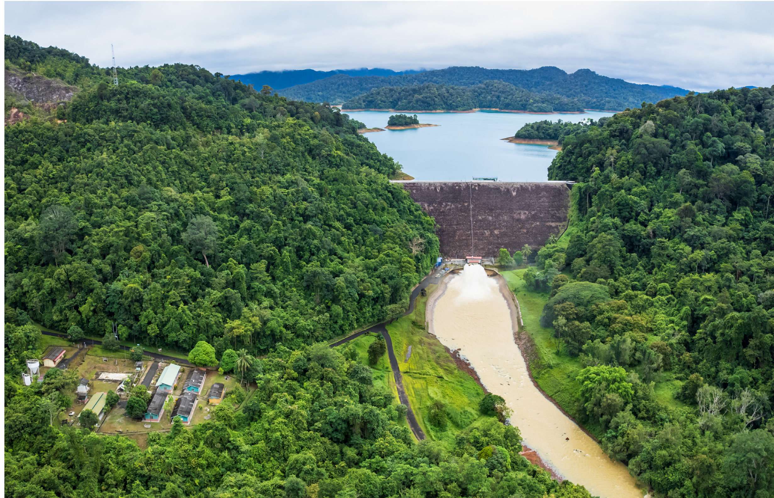
Pedu Dam, a major rock-fill embankment in northern Kedah, creates the expansive Pedu Lake that supplies vital water for Malaysia's Rice Bowl. The reservoir supports irrigation, strengthens regional water security, and anchors the forested landscapes linked to the Ulu Muda watershed. (Photo courtesy of LSANK, Malaysia)
