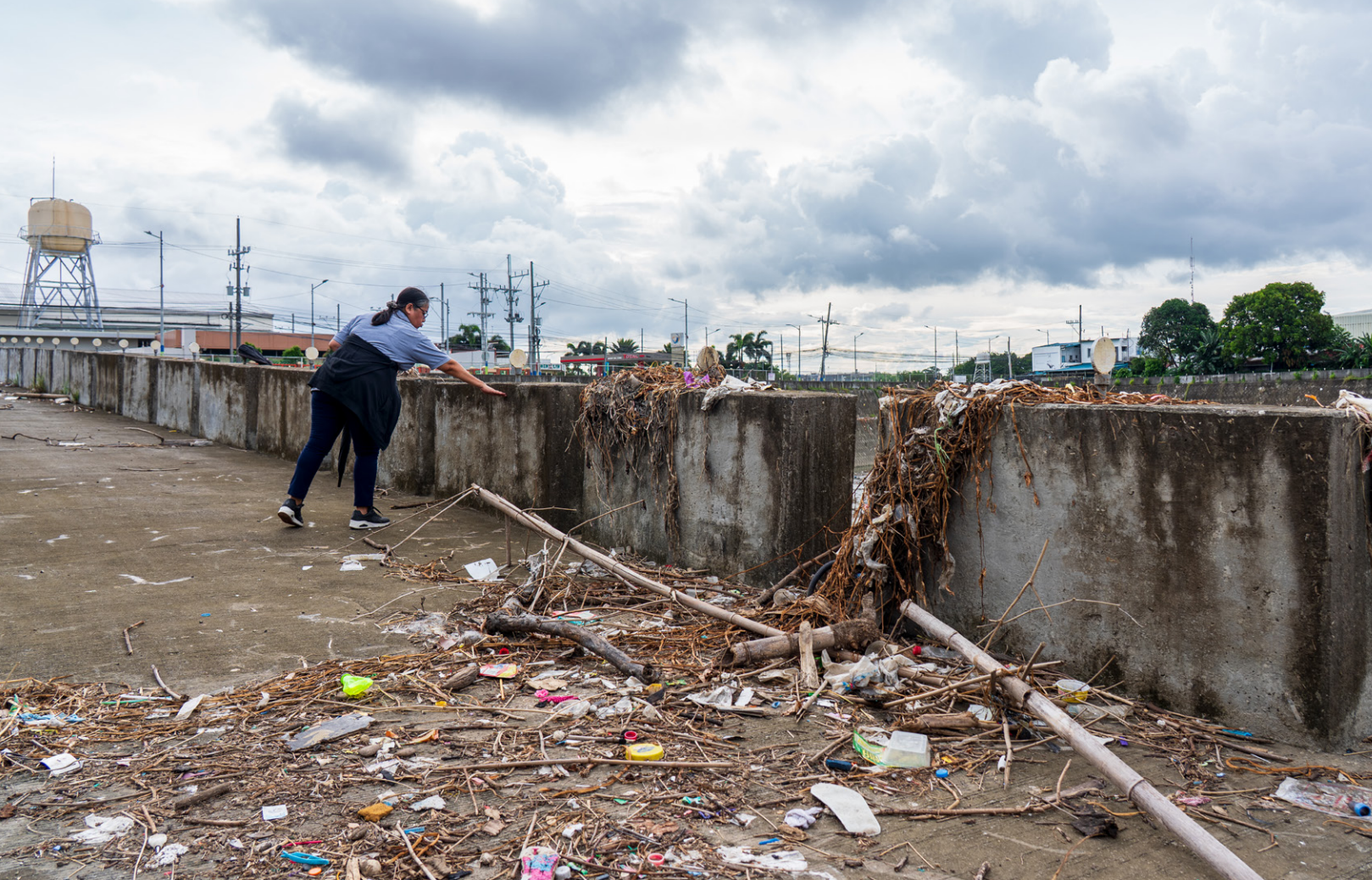
Trash along the concrete walls of the Bacoor Retarding Basin marks the water level during heavy rains. (Photo by Orange Omengan/PEMSEA)
