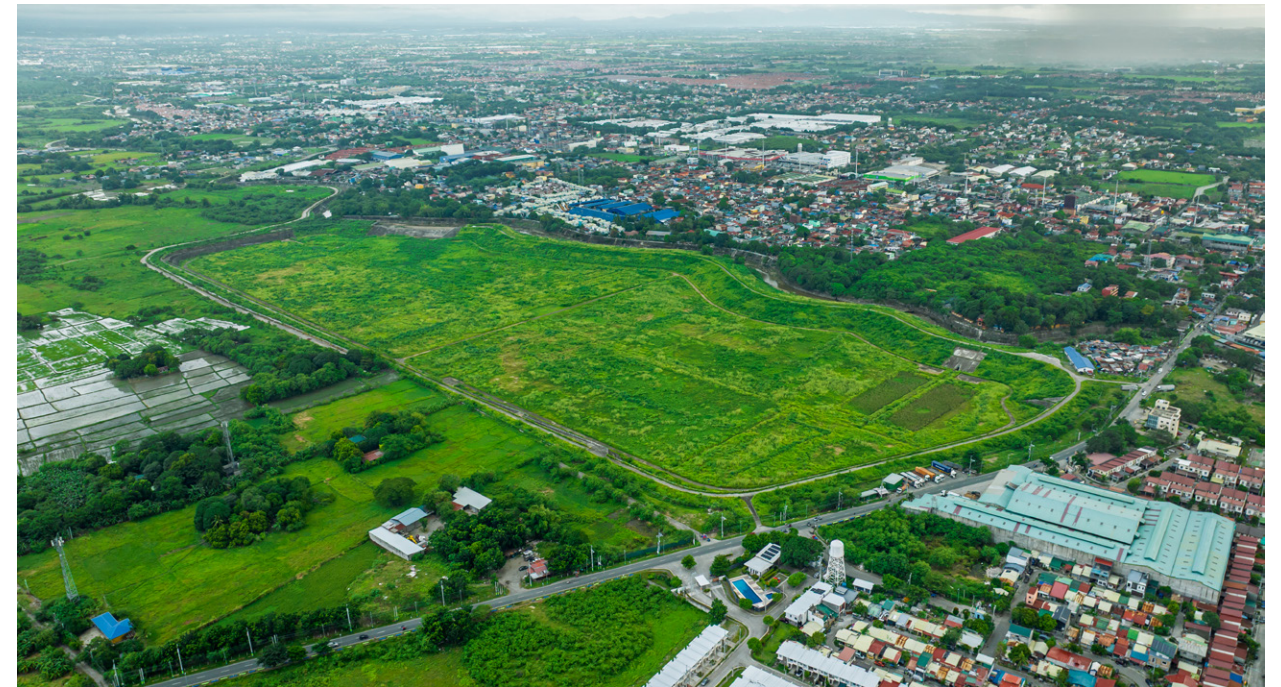
The Imus Retarding Basin in Barangay Anabu 1-A in Imus City, Cavite. (Photo courtesy of the Provincial Government of Cavite)
