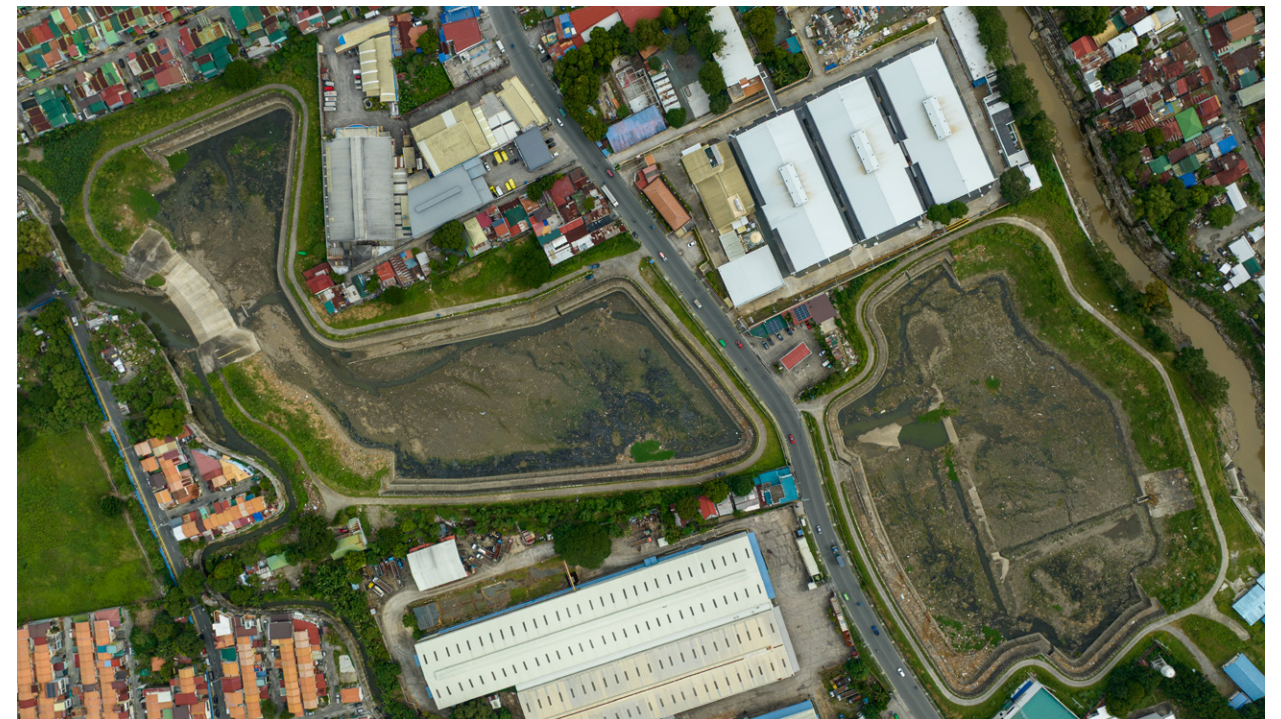
The two storage ponds of the Bacoor Retarding Basin in Barangay Buhay na Tubig, Imus City, Cavite. (Photo courtesy of the Provincial Government of Cavite)
