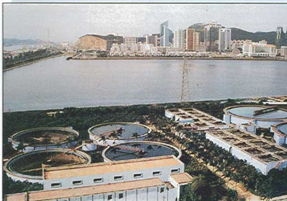
Sewage Treatment Plant, Yuan Dang Lake, Xiamen, China.
