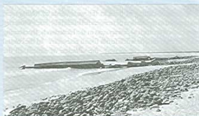
Concrete groins constructed along the shoreline for beach protection against swell.
