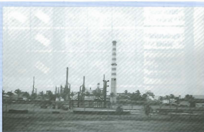
The Caltex refinery in Batangas Bay area, Philippines.
