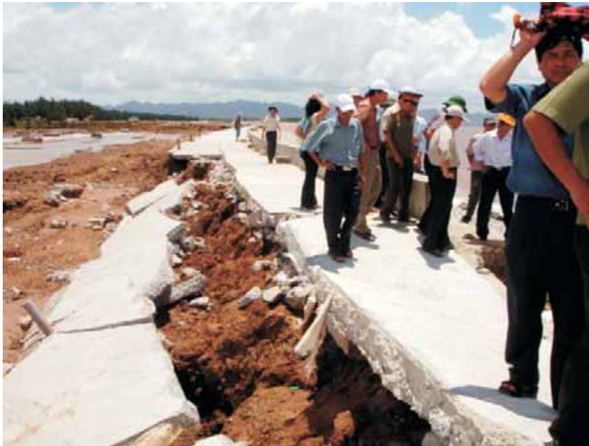
Damage caused by the Damrey Typhoon in July 2005 to Hai Hau in Nam Dinh Province.
