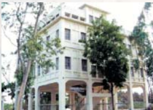
Cyclone shelter in Chittagong, Bangladesh.
