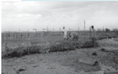
Photo 1. Brush fascine as wave breaker.
