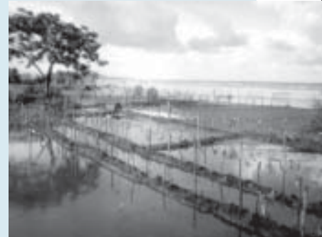
Photo 4. Vegetated coir logs installed on site.
