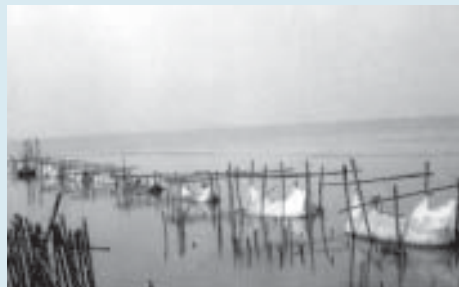
Photo 2. Mud bags as wave breaker.
