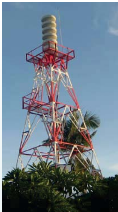
A siren tower for a tsunami early warning system
