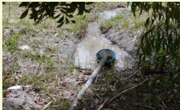
Wastewater discharging onto the ground surface.
