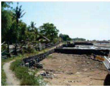
Eroded beaches in Sanur before rehabilitation.
