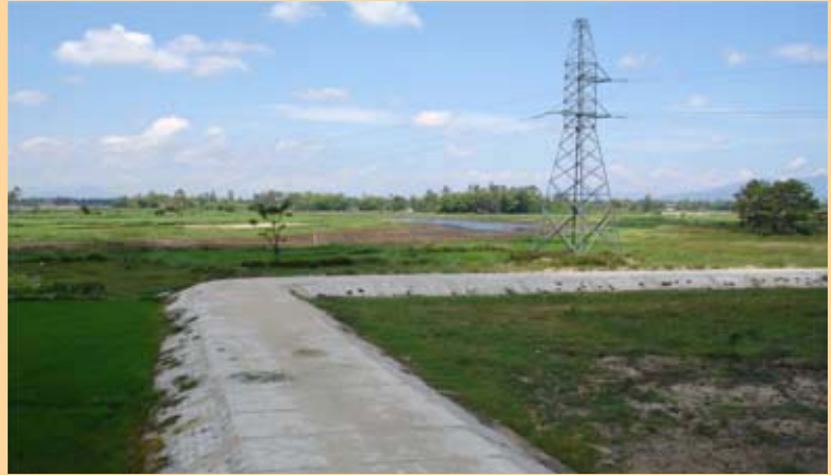
Dike system to prevent saltwater intrusion.
