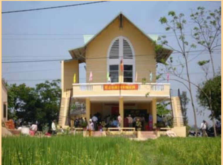
Multipurpose shelter house for typhoons and floods.
