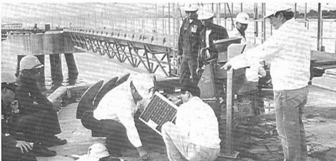
Korean experts installing tidal monitoring equipment at the Batangas Bay
