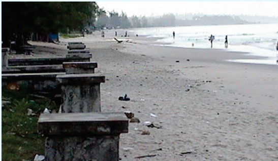
Photo 9. Concrete posts within the easement and buffer zones were established on public land in the beach.
