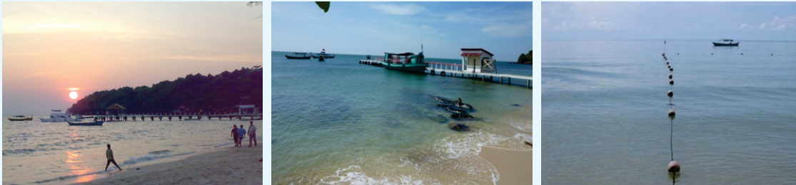
Photos 6–7. A pier was established for vessel anchorage and as an embarkation point.
