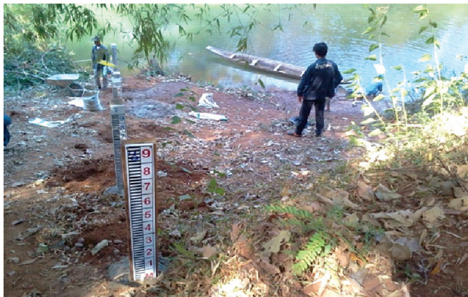
Figure 8. Installation of gauges for water monitoring.
