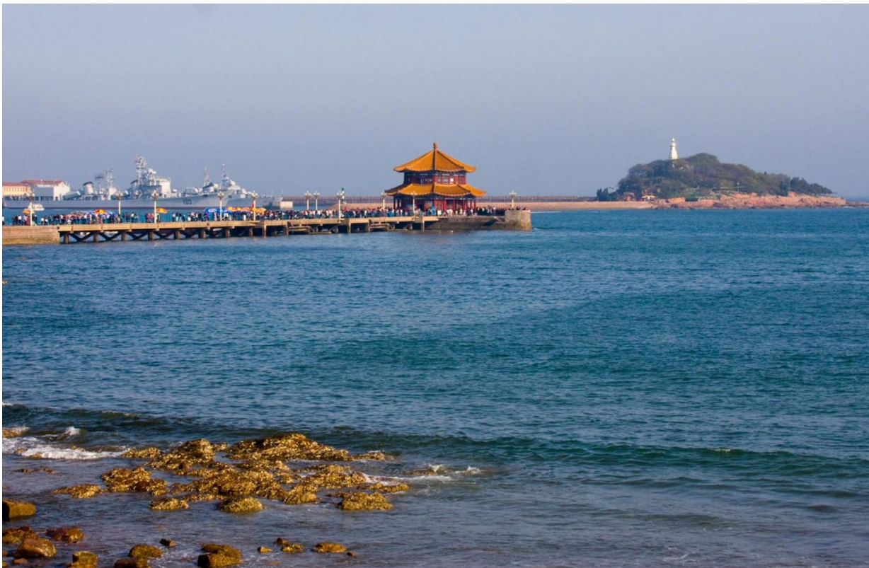
Qingdao Pier, China (Photo by M. Ebarvia)
