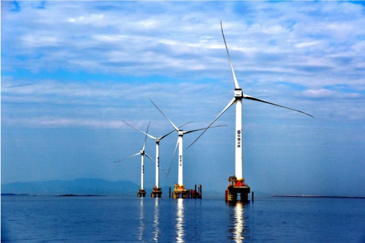
Offshore wind power project of China Three Gorges Corp (CTG) in Fujian Province (Photo courtesy of CTG)
