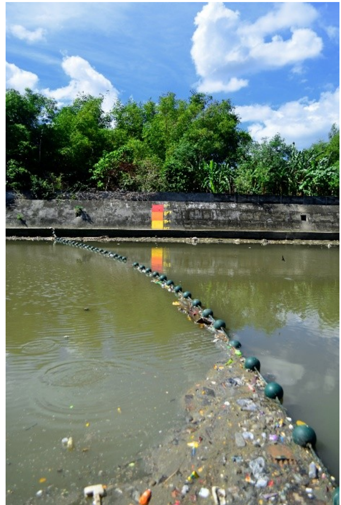
A trash boom helps trap and collect floating riverine debris in Bacoor.
