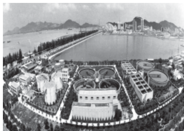
Sewage treatment facilities in Xiamen
