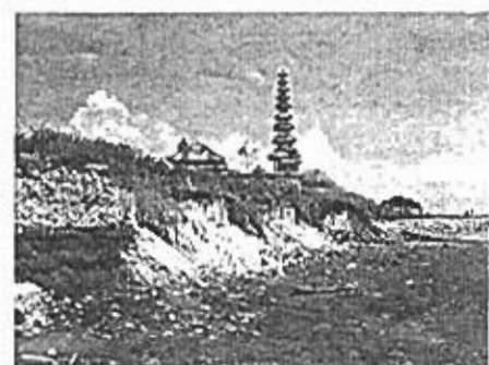
Photo 23. Beach erosion in Padang Galak.
