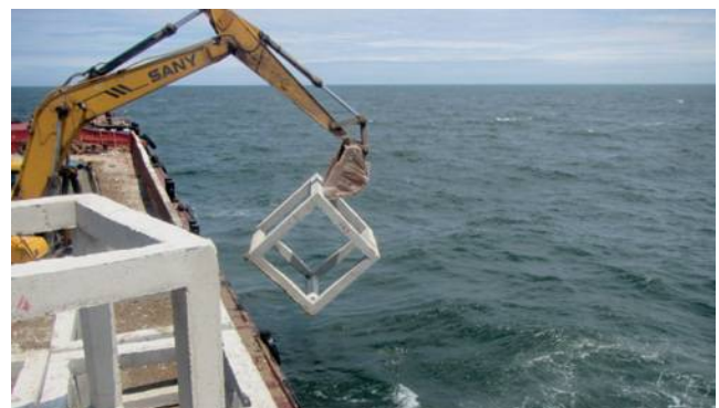
Ecosystem-based Fisheries in Lianyungang: deployment of artificial reefs.
