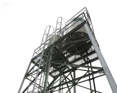
Tanks for reuse of treated wastewater
