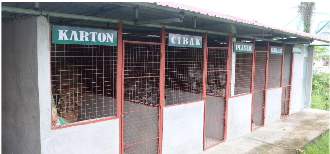
Waste segregation—shown here in San Jose, Tagaytay—is key to proper solid waste management.
