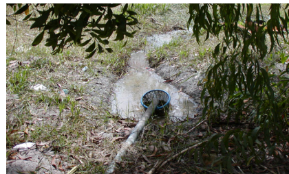
Wastewater discharging onto the ground surface.
