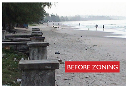
Concrete posts within the easement and buffer zones were established on public lands in the beach.
