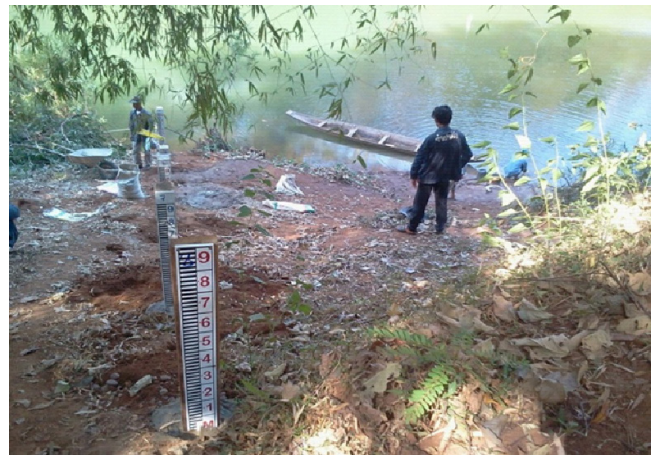
Installation of gauges for water monitoring.
